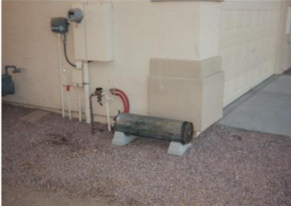
This picture represents the portable exchange tank cover resting over the portable exchange tank (which is laying on the cradles).
